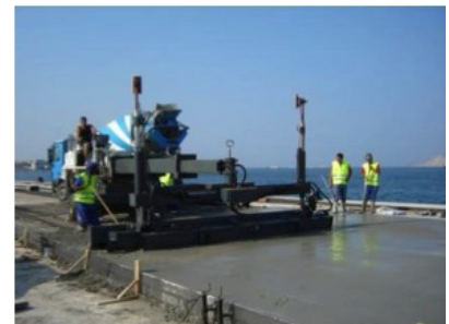
Figure 1. Layering of ready-mixed concrete for the construction of heavy duty surfaces.
