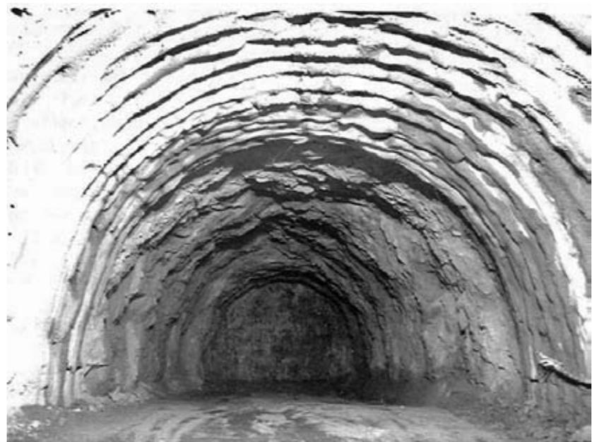
**Figure 3. Overprofiled (overbreak) tunnel excavation and tunnel supporting by tunneling in karst** (Source: TUNEL MALA KAPELA – NAJDUŽI TUNEL U HRVATSKOJ), GRAĐEVINAR 56 (2004) 1)
